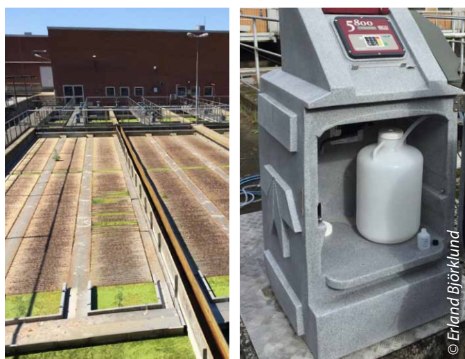
Figure 1. Sampling points of treated wastewater at the outlet of Kristianstad WWTP (1a, left) and Tollarp WWTP (1b, right).
